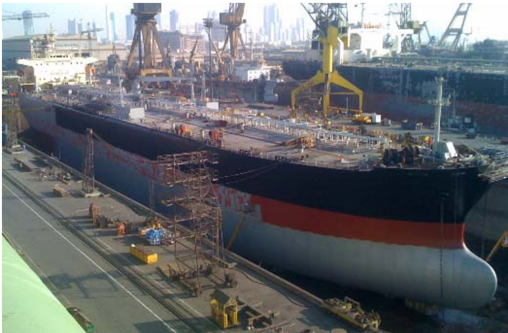
The CE EXPRESS seen in Dubai Drydocks undergoing drydocking repairs
