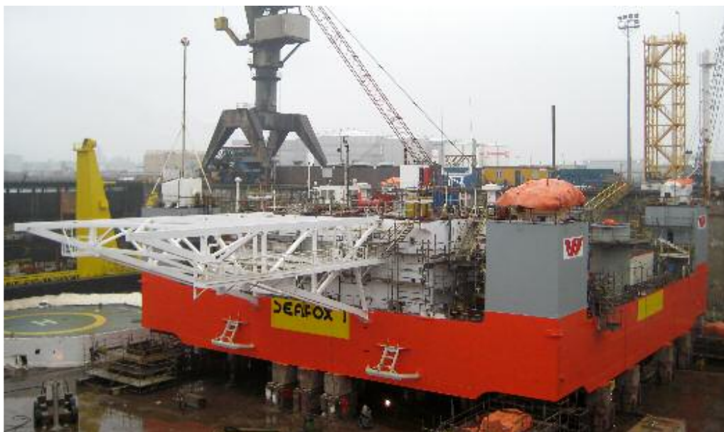
The SEAFOX 1 seen in drydock at the Keppel Verolme yard in Rotterdam
